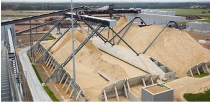
Figure 17 - 'A' Frame type FIFO Stackers Reclaimer (Valmet)
